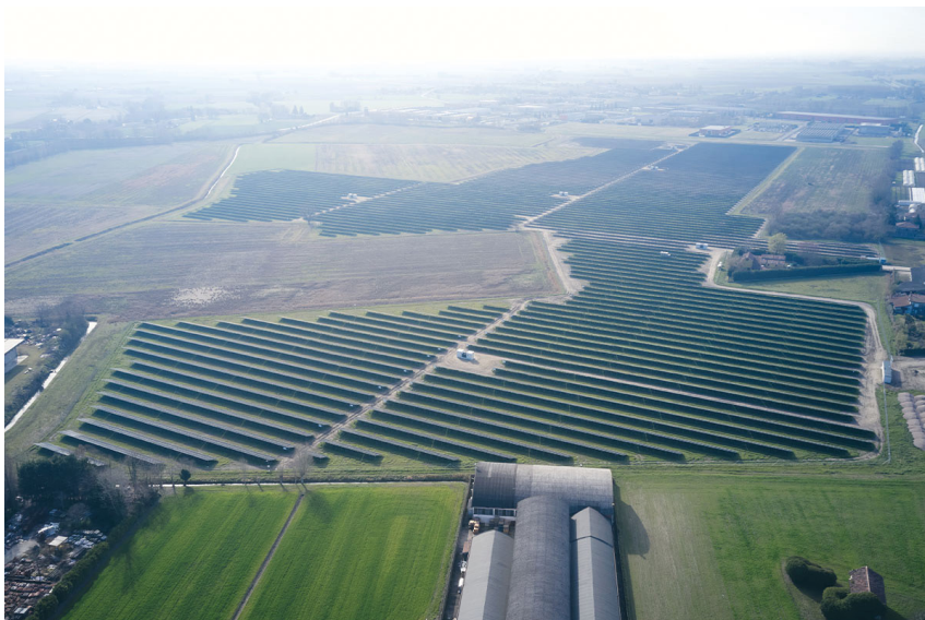
CHART 17 – PHOTOVOLTAIC SYSTEM AT BADIA POLESINE
